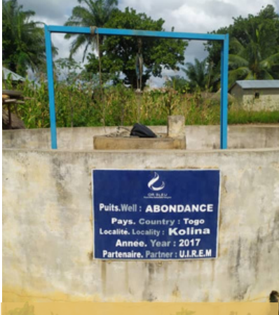
Puits - Village Kolina Inauguration le 08/10/2017
