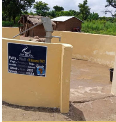
Puits - Village Soukounde Inauguration le 31/08/2020
