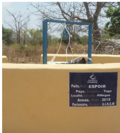
Puits - Village Adbegue Inauguration le 05/03/2018
