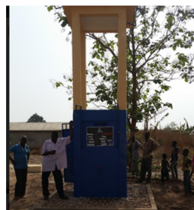
Forage - Village Diliko 2 Inauguration le 25/02/2019
