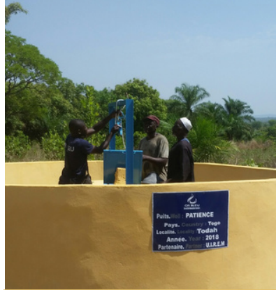
Puits - Village Todah Inauguration le 11/03/2018
