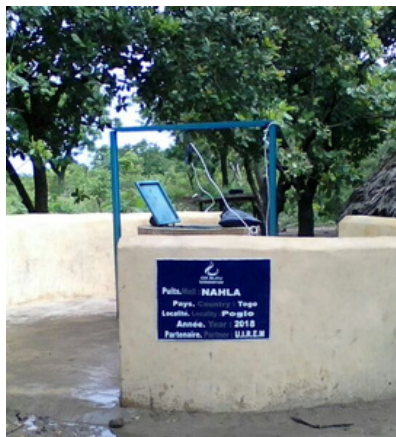
Puits - Village Pogolo Inauguration le 30/04/2018
