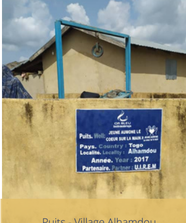
Puits - Village Alhamdou Inauguration le 02/12/2017
