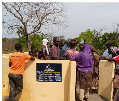
Puits - Village Karkassou Inauguration le 25/04/2021
