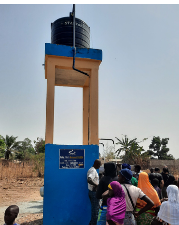
Forage - Village Yomaboua Inauguration le 25/01/2022
