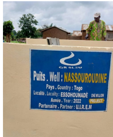
Forage - Village Essohounade Inauguration le 03/08/2022
